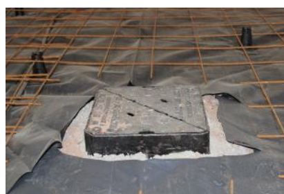
Installation uses standard building materials
